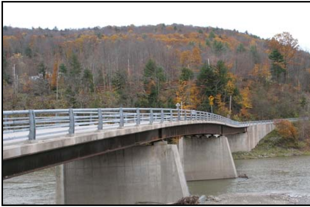
Lordville Bridge and Manchester Township Ridge Line
